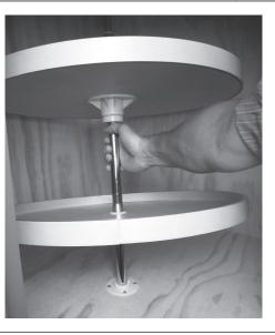
Turning a shelf upside down, attach the Shelf Hub with four (4) - #6 x 1/2" Pan Head Phillips Wood Screws in the center of the mounting slots as shown. Turning shelf back over push the Shelf Collar into the top of the shelf until flush. Repeat with second shelf.
